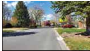
Exhibit 27. Existing sidewalk gaps on Division Street south of Bath Street would be address by project WZ-11
