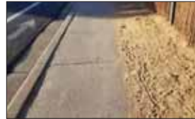
Exhibit 32. It is recommended that sidewalks on Saliman Road (WZ-28) be widened.
