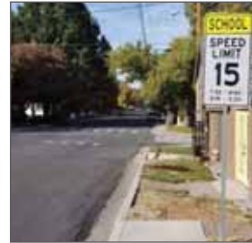
Exhibit 6. Sidewalk gap on Thompson Street in the Bordewich-Bray School Speed Zone
