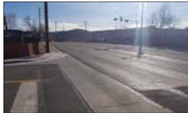
Exhibit 24. Fairview Drive at Walker Drive, looking south (CS-3)
